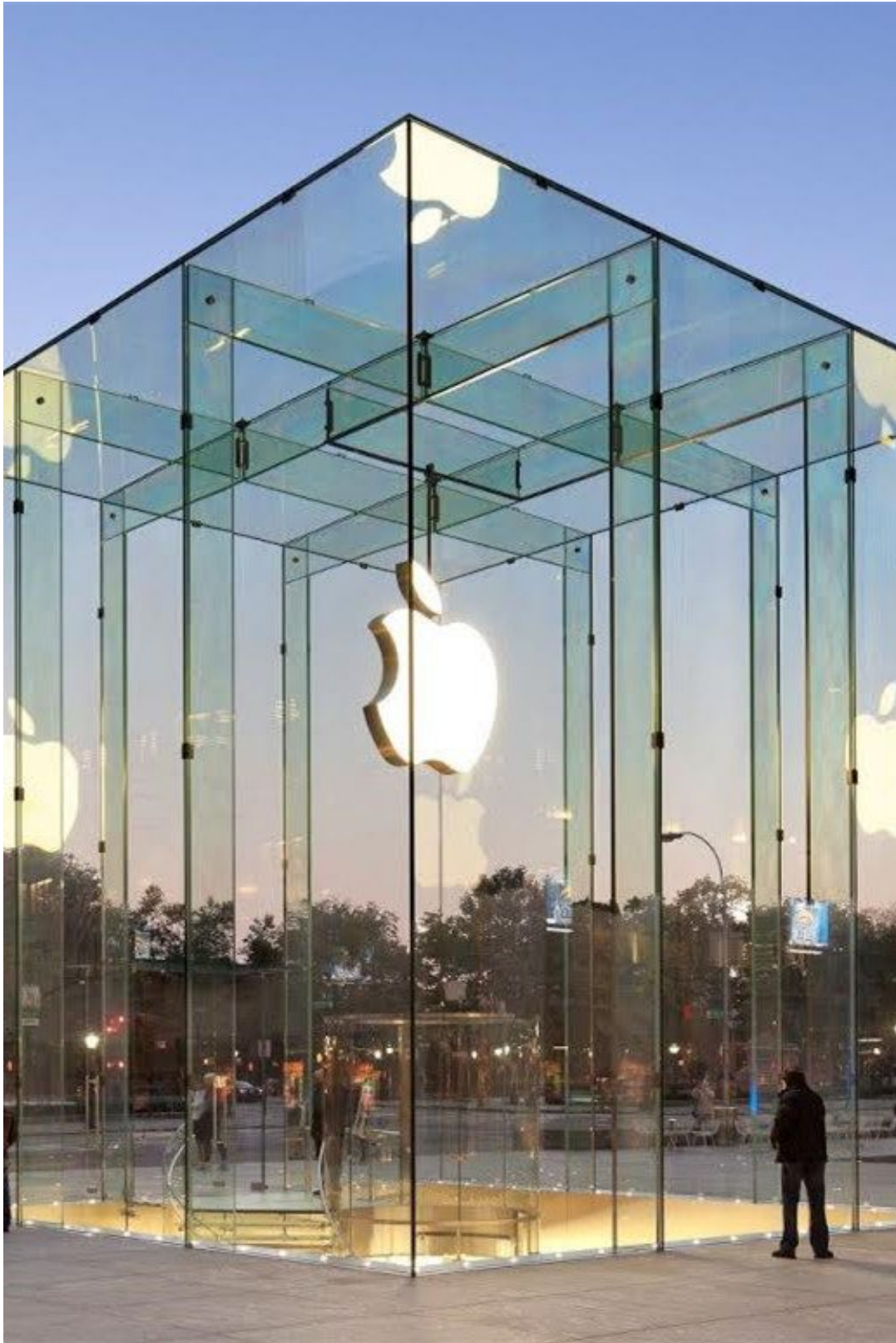
laminated glass fin for curtain wall/ facade
