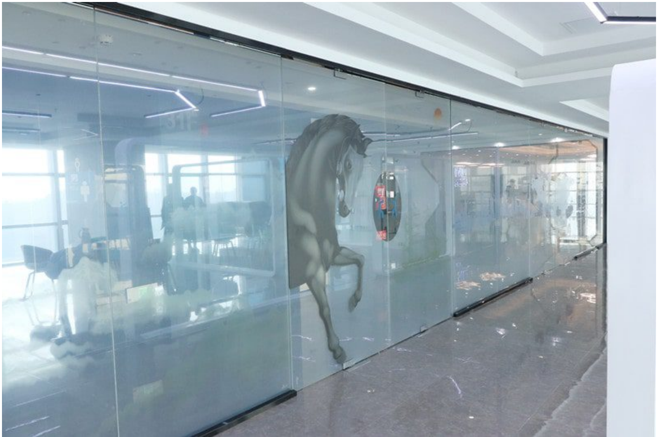
smart glass electric privacy glass partition ON
