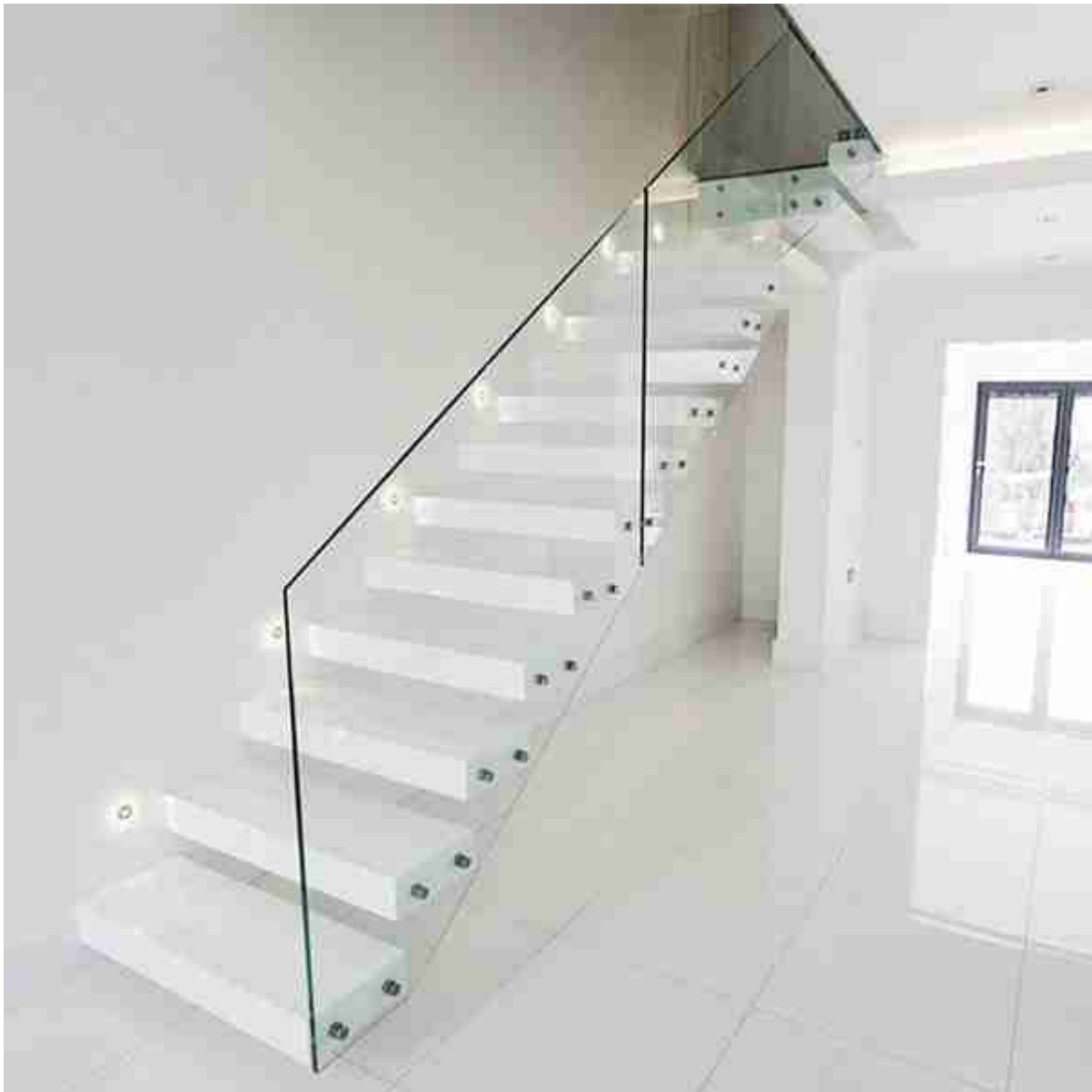
Frameless bolts tempered laminated glass railing staircase:
