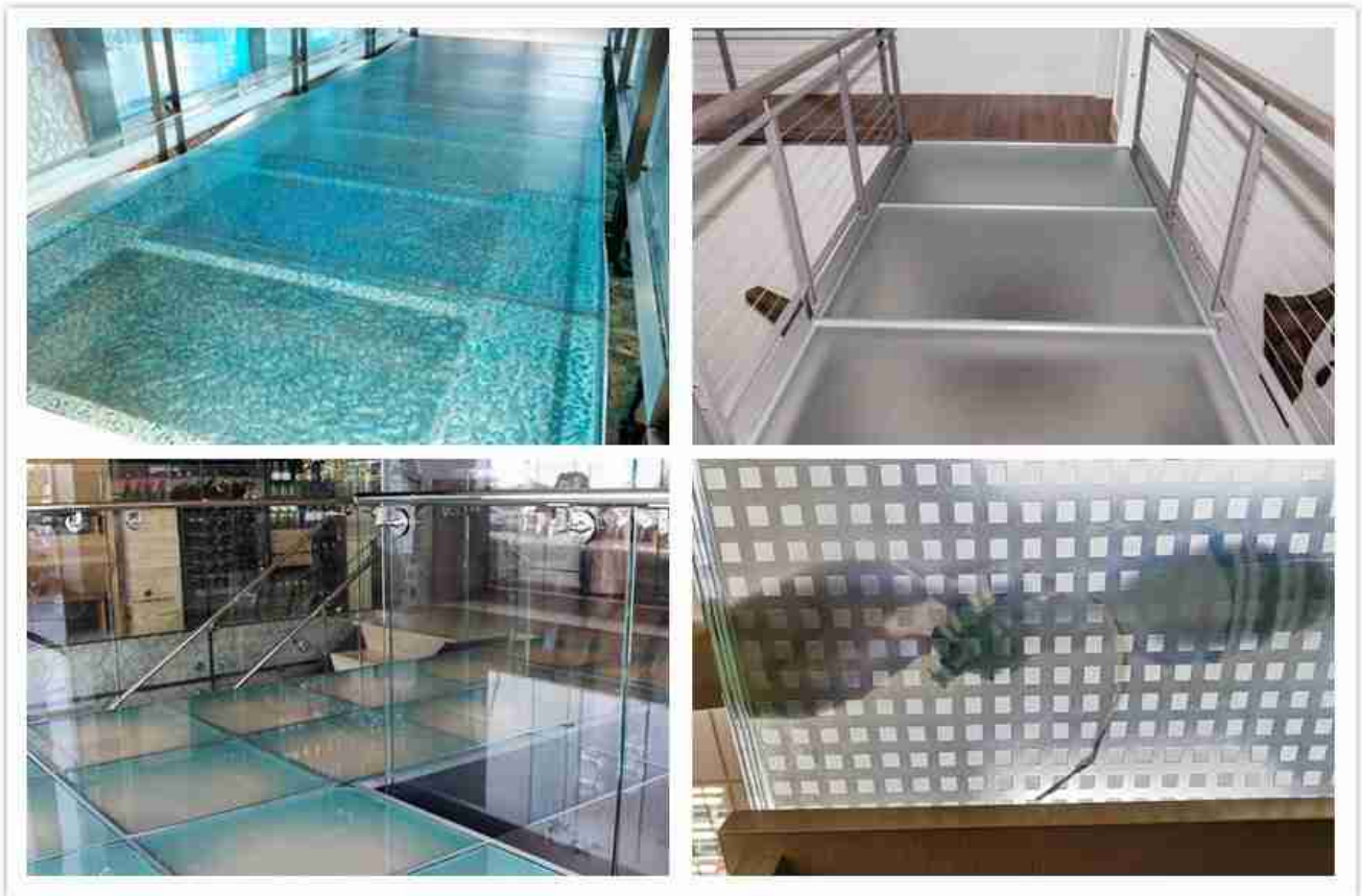
Different kinds of anti-slip patterns for laminated glass flooring
