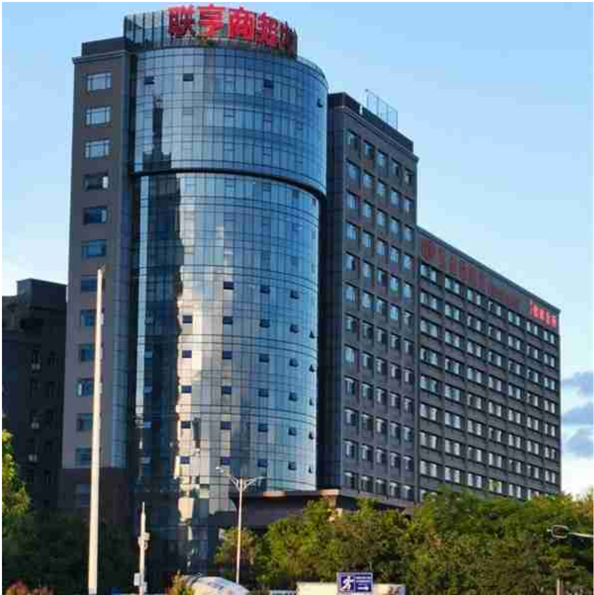
Double glass facade
