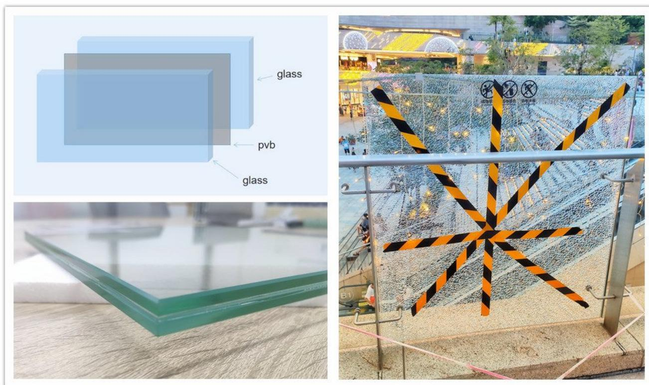
Tempered laminated glass, when one piece breaks, the other panel and the PVB will glue the glass together bidding time for a replacement.
