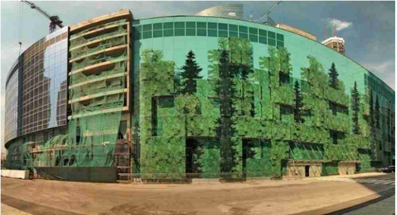
Digital ceramic glass printing for curtain wall
