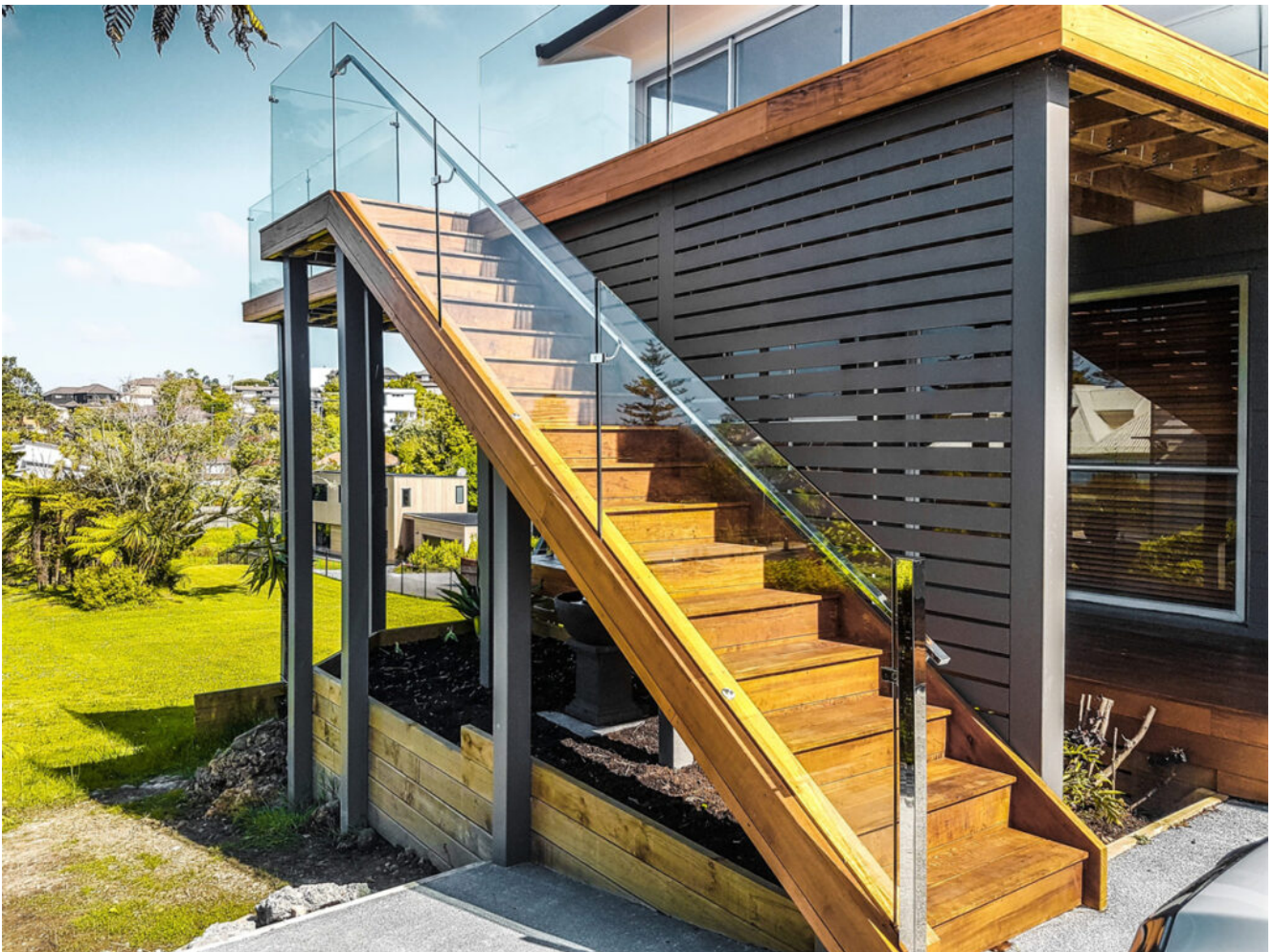
8+8mm clear tempered laminated for frameless balustrade
