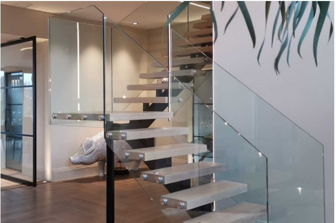
8+8mm clear tempered laminated for frameless balustrade
