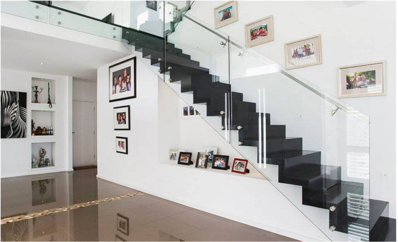
8+8mm clear tempered laminated for frameless balustrade
