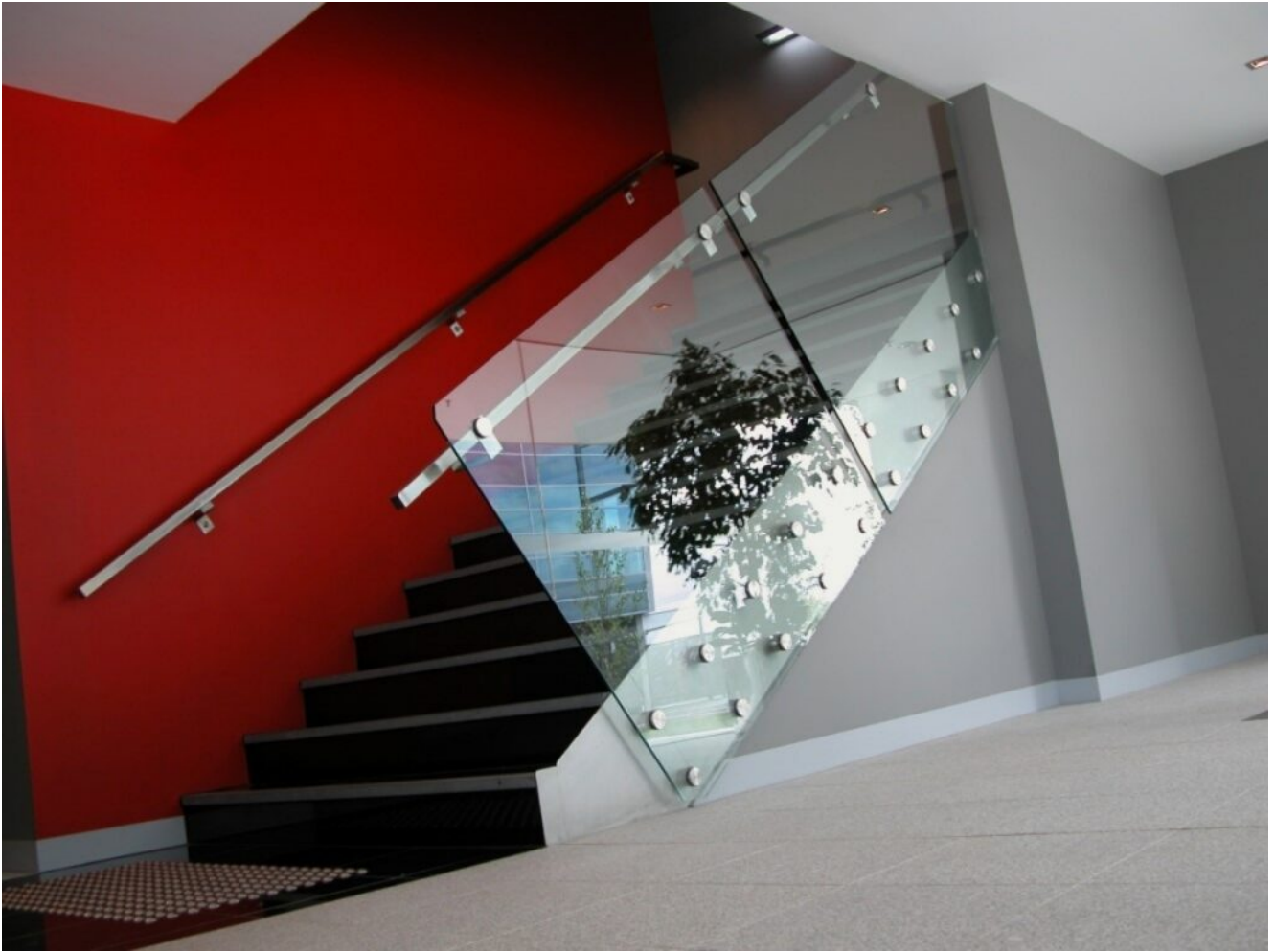
8+8mm clear tempered laminated for frameless balustrade
