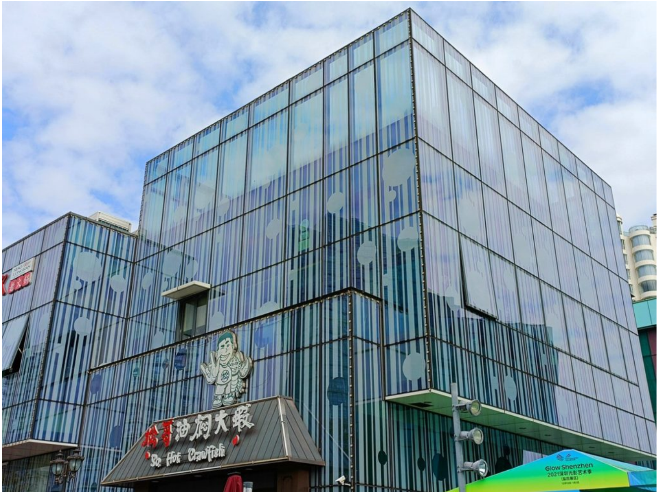
silk screen printing double insulated glass panels for facade
