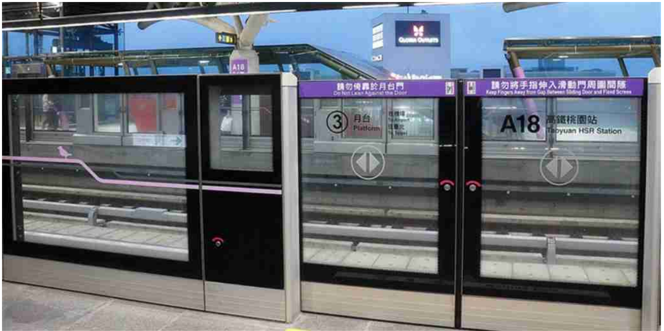
12mm toughened gradient design ceramic frit glass for metro platform glass door
