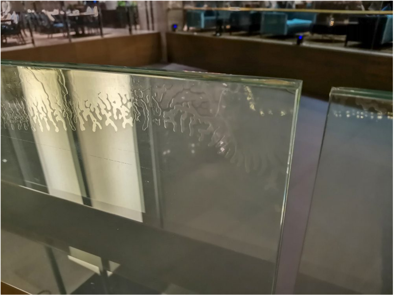
PVB laminated glass delamination
