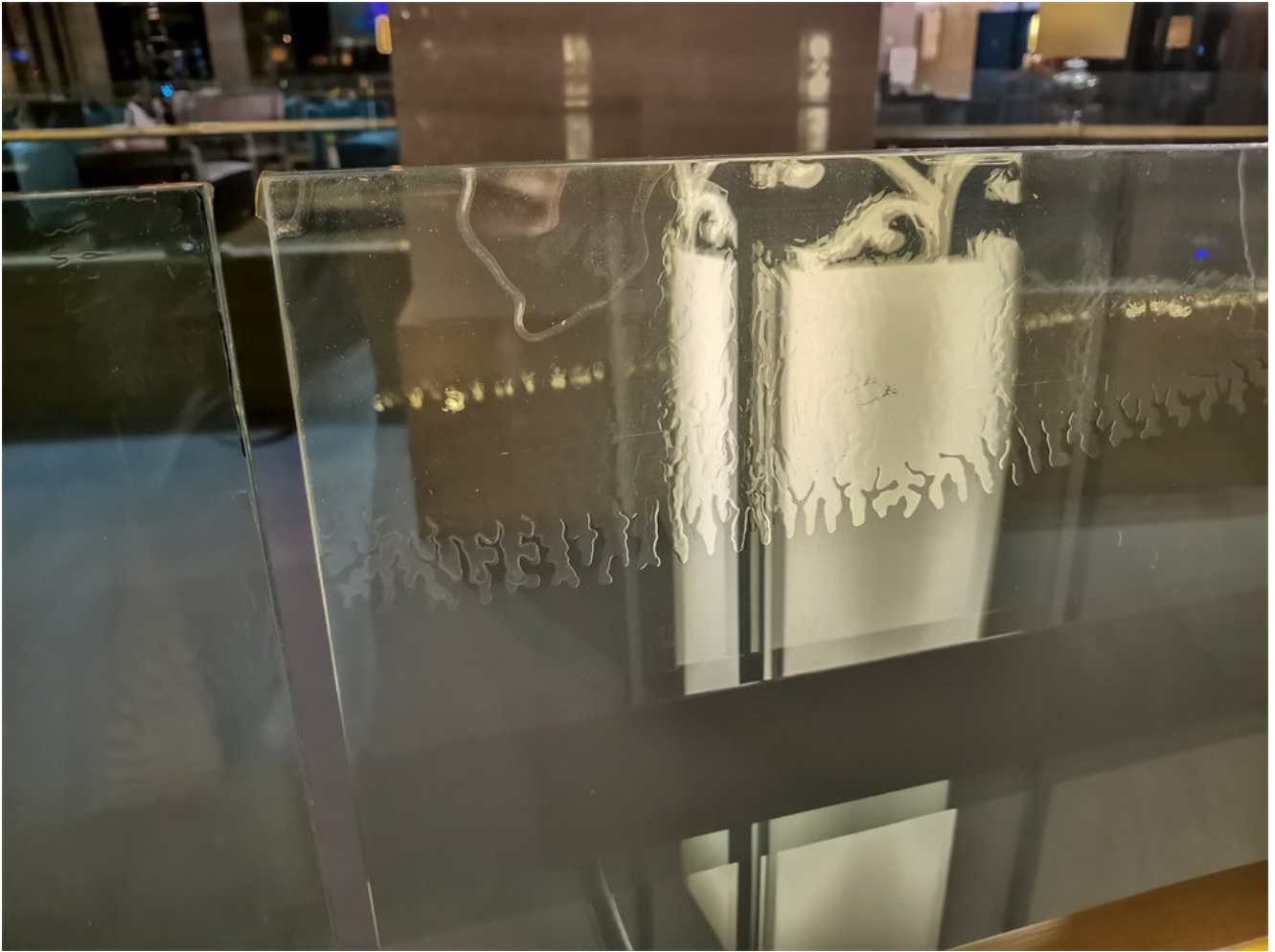
PVB laminated glass delamination
