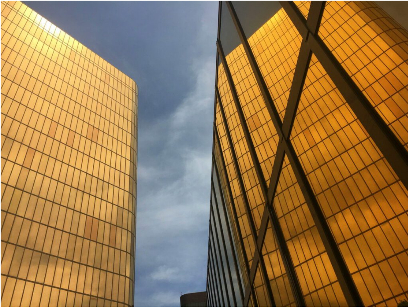
golden Low- E double glazed sealed units facade windows
