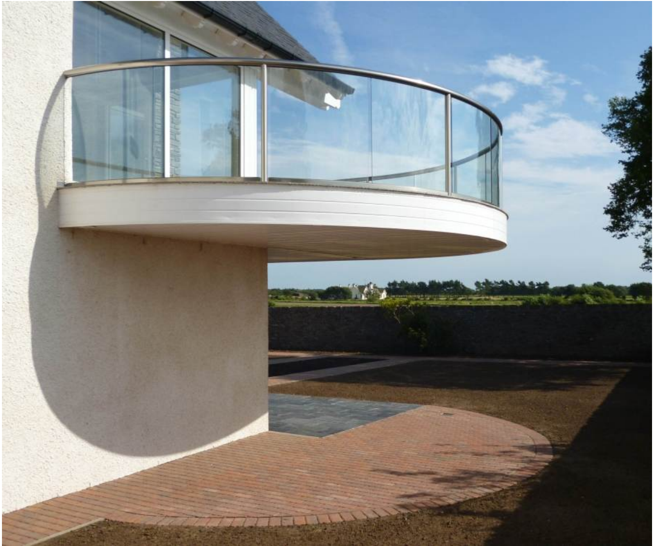
curved laminated glass for balcony glass railing
